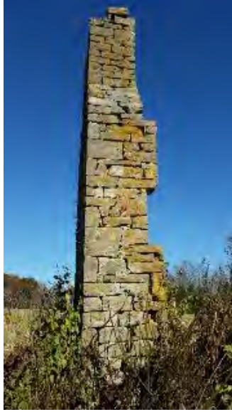
Mordeci Collins pioneer dry stacked fire place
